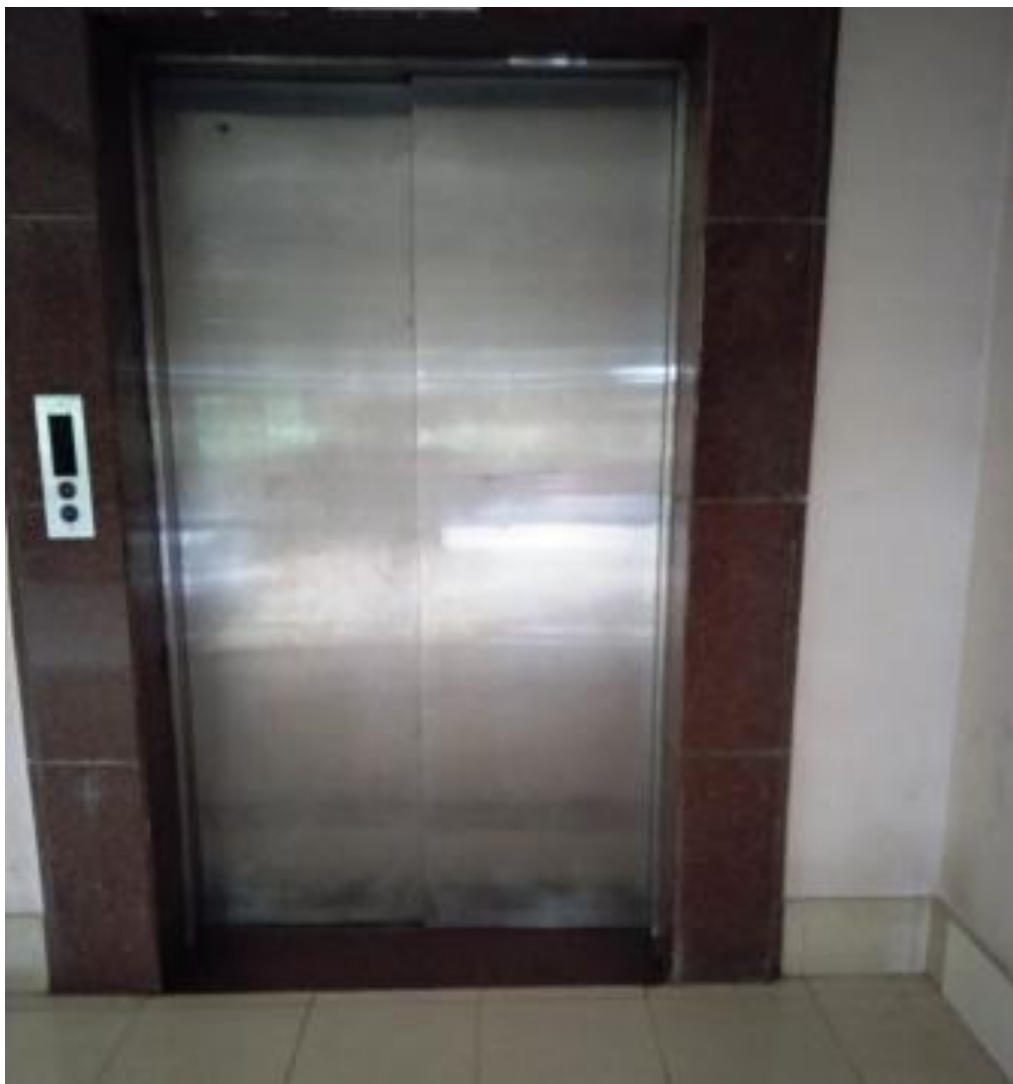
Photograph Showing Lift provision at the College
